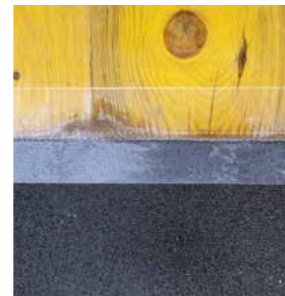
The bearing tape is double perforated. One side sticks to the formwork board, the other sticks to the ceiling bearing.
