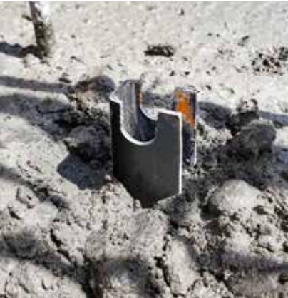
Insert the U-profile into fresh concrete.
