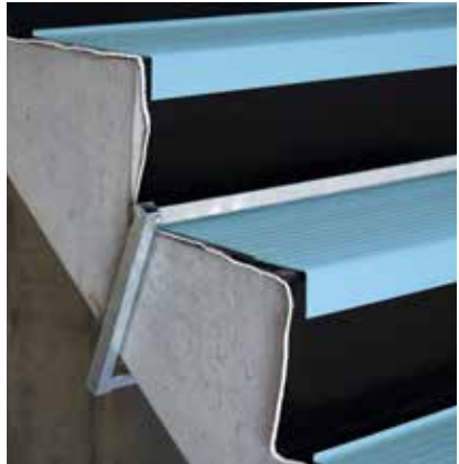
Attaching the stair protection angle with brackets.
