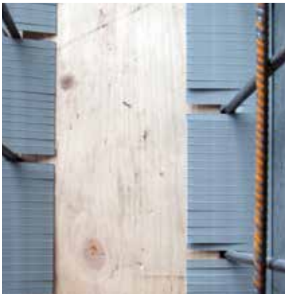
ferrofix comb also works on wall sections.
