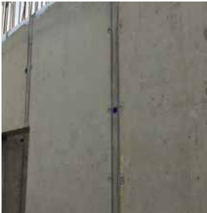
Patch between formwork elements
