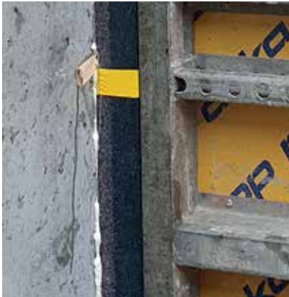
Patch between formwork elements
