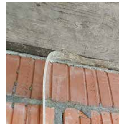
Tear off the bearing tape after stripping
