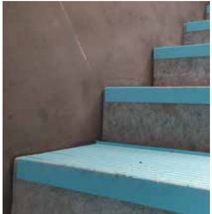
Stair protection angle attached with a square timber.
