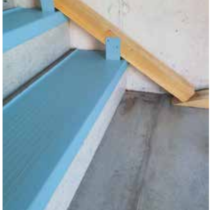
Stair protection angle attached with a square timber.
