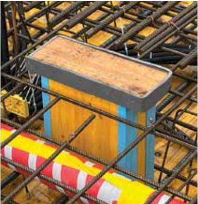
Lift out formwork boards individually
